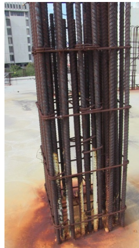
Figure 9: Oxidation at Base of Column on Second Floor Slab (Photo log Image #126)
