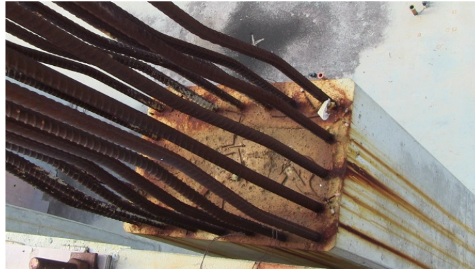
Figure 8: Oxidation on Top of Unfinished Columns (Photo log Image #127)
