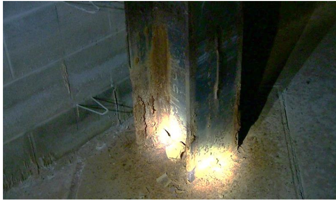
Figure 2: Area G Basement Column Oxidation (Photo log Image #214)
