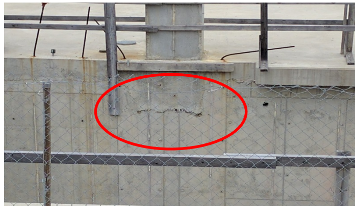
Figure 7: South Open Area to Small Basement Chamber, Crack Close-Up
